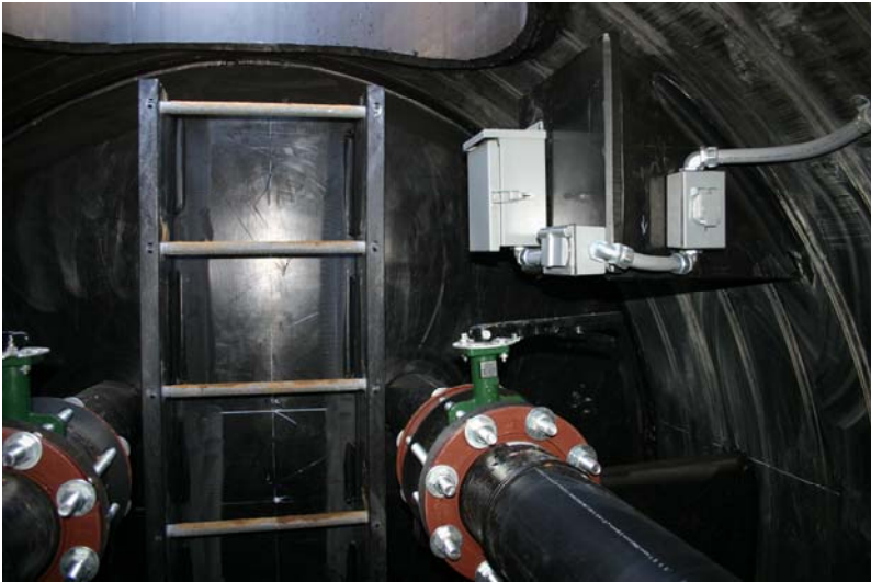
Photograph #8: Geothermal Vault Ladder
