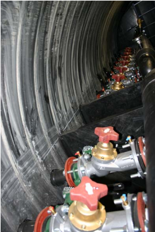
Photograph #7: Geothermal Vault Wall Surface
