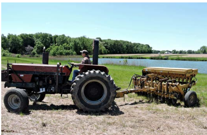
Top: A recently installed wetland in a soy bean field. Left: A contractor plants grass and wildflowers in a newly created buffer.
